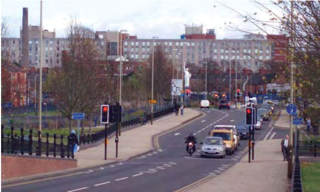
Photo 2.1: Upperton Road Viaduct Scheme
