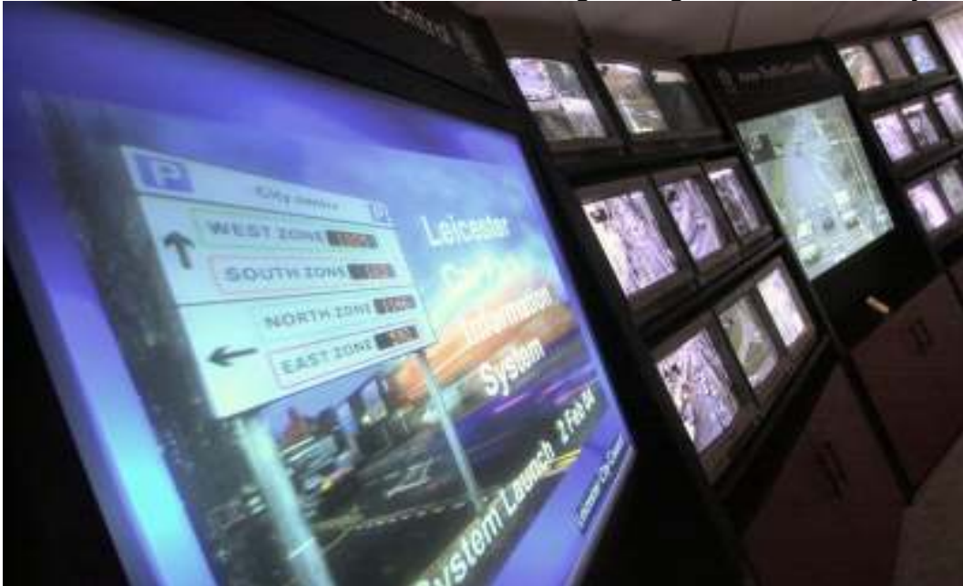
Car Park Variable Message Signs and Screens in the Urban Traffic Management Centre
