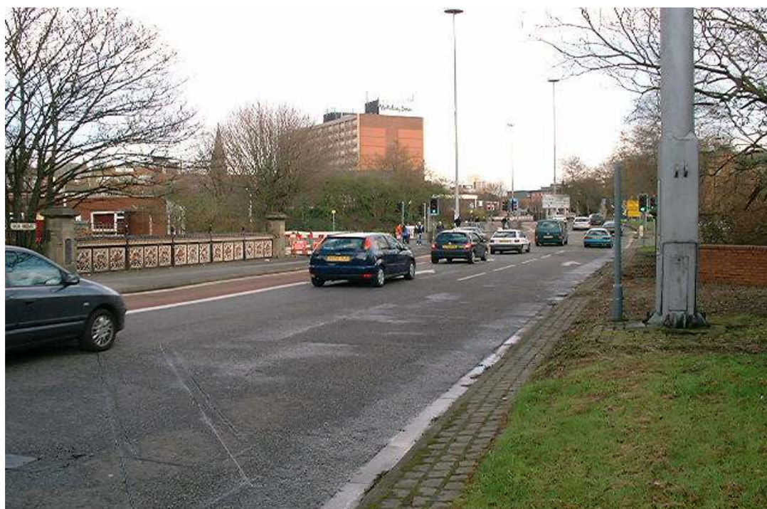
(Old Bow Bridge (No.4): Major maintenance works carried out in 2009)
