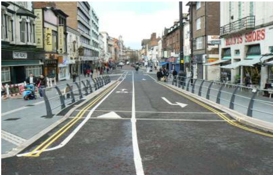
New carriageway/footway construction at Granby Street (2010)
