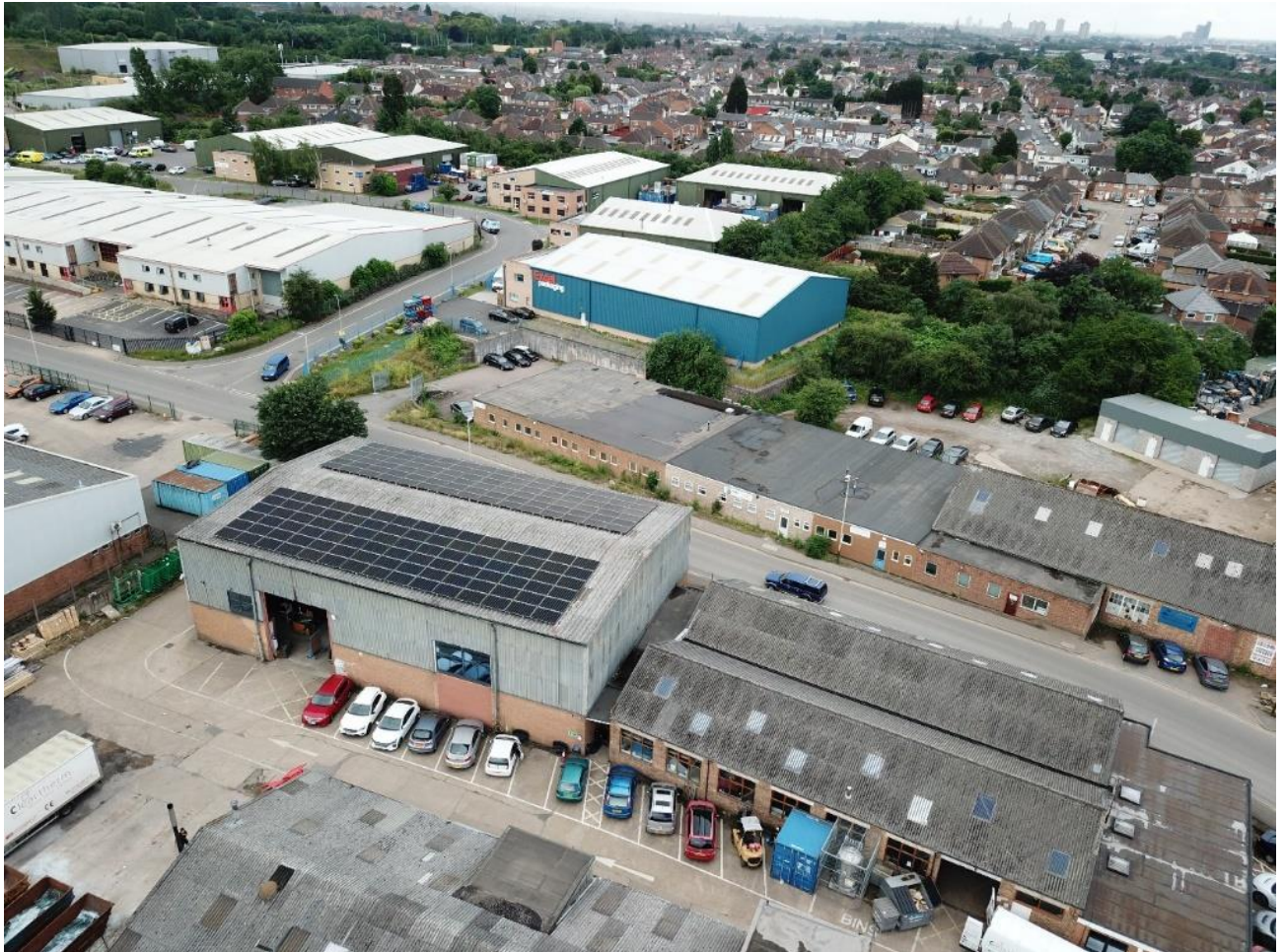
Drone photo of the new solar panels on the warehouse roof - Photograph © Cleartherm Glass Sealed Units Ltd
