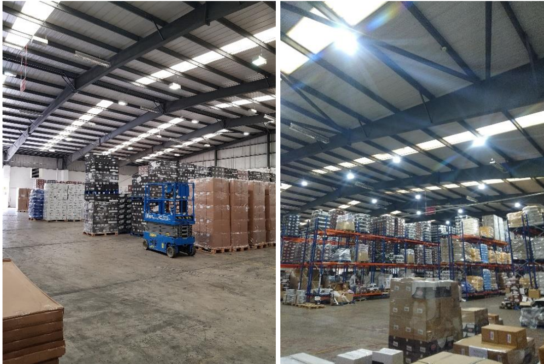
Before (left) and after (right) replacing the lighting with energy-efficient LEDs
