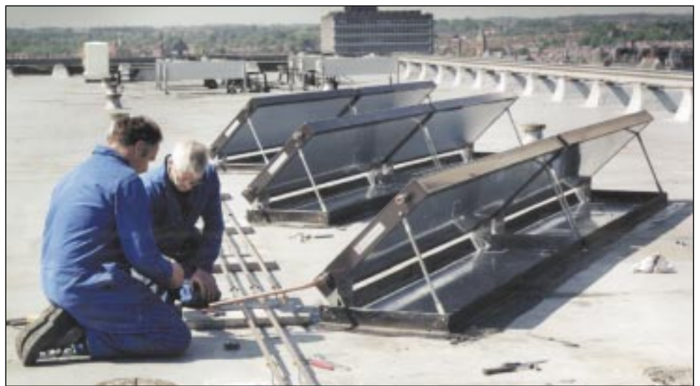
Installation of six flat-plate collectors on the roof of B Block
