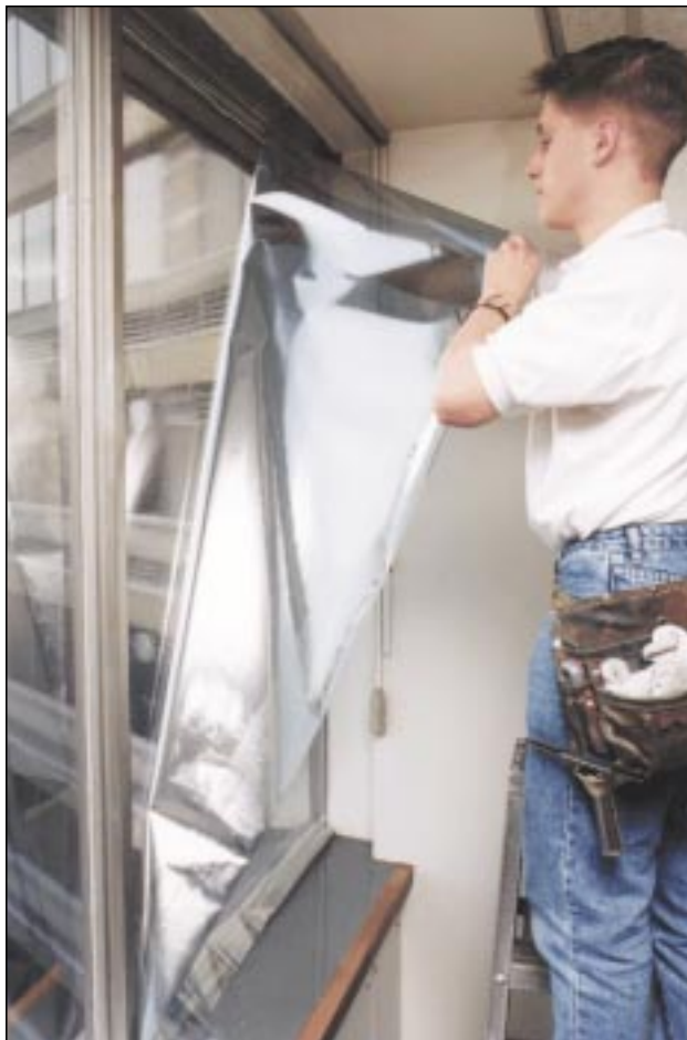
Installation of film
