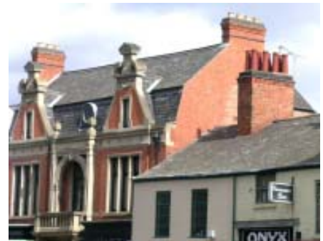
Roof lines are important: at 73 Church Gate a Mansard type roof clad in Welsh slate adds much distinction.
