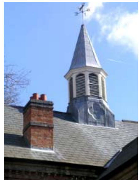
The timber and lead covered cupola to the roof of the Great Meeting Schoolrooms supports a fine weathervane.
