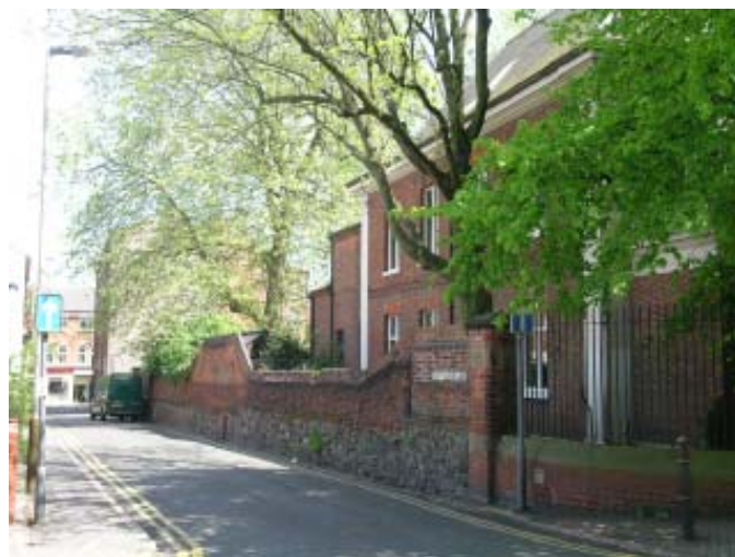
Butt Close Lane: the 18th century boundary brick wall is constructed on the remains of an earlier stone rubble wall.
