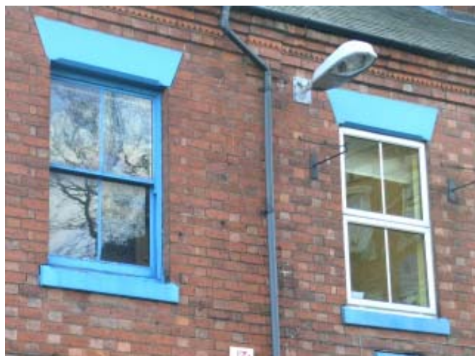
Two different types of window from the same property: the window to the right has been replaced in uPVC. The window to the left is an original timber sliding sash and is complete with Victorian glass incorporating elegant vertical glazing bars.
