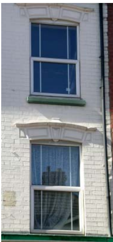
Windows are like the eyes on a human face - they are a point of contact that draw our attention and are an integral part of the architecture of a building. Their alteration or removal can reduce the value of a property both visually, historically and financially. These two examples from within the conservation area show windows that have been replaced with unsympathetic uPVC material.
