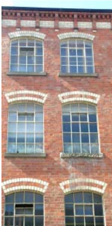
Most of the architectural detailing including polychrome brickwork and original cast iron windows still survive to the upper floors of factory premises at 74-76 Church Gate.
