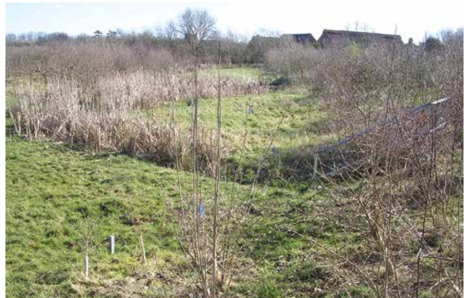
Glenfrith housing area; a necklace of water retention areas; good for stormwater but not so good for wildlife and wetland benefit.
