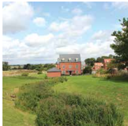
Swale; in new housing area shows the amenity value of the system
