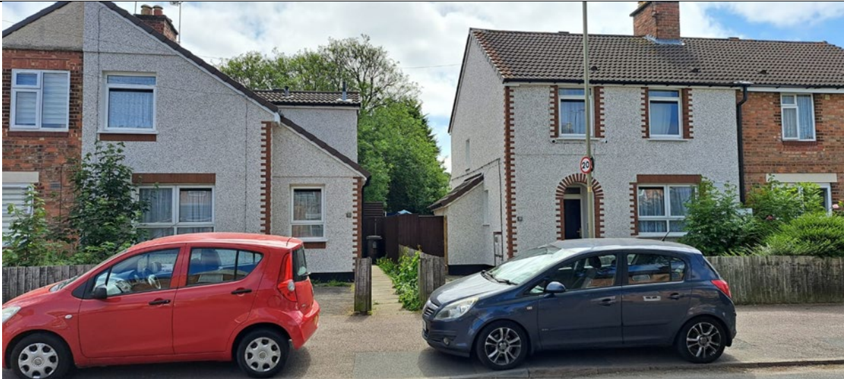
Two examples of EWI finished in pebble dash render with carefully positioned brick slips to retain character/detailing of the area
