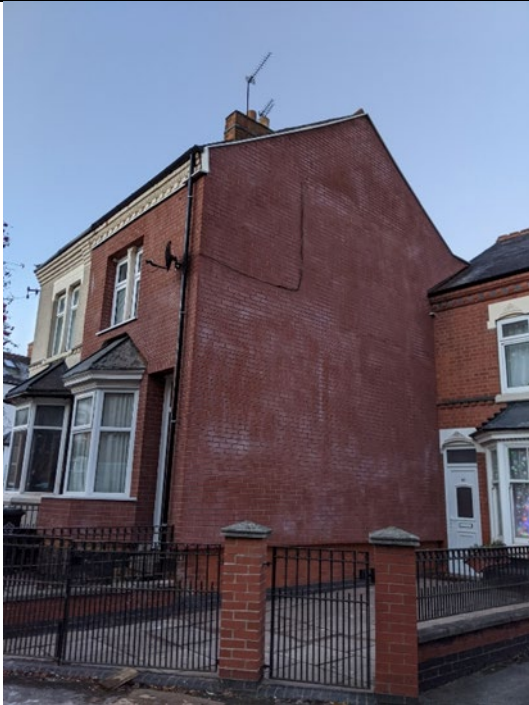
EWI finished with brick slips in a mixed hue finish with eaves detailing replicated.
