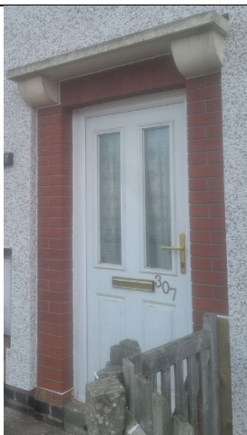
Brick slips for door surround
