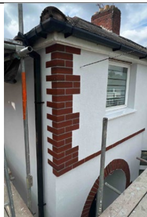
Brick slips for corner detailing
