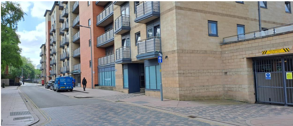
Blackbird Fields (Barratt Homes) Highway works New access
