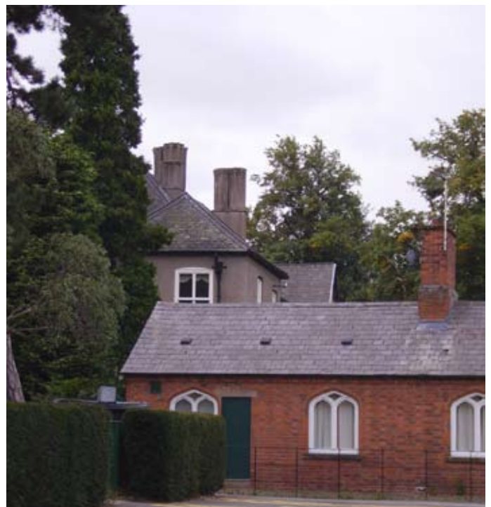
Gothic-style windows to the former stable-block at Aylestone Hall.
