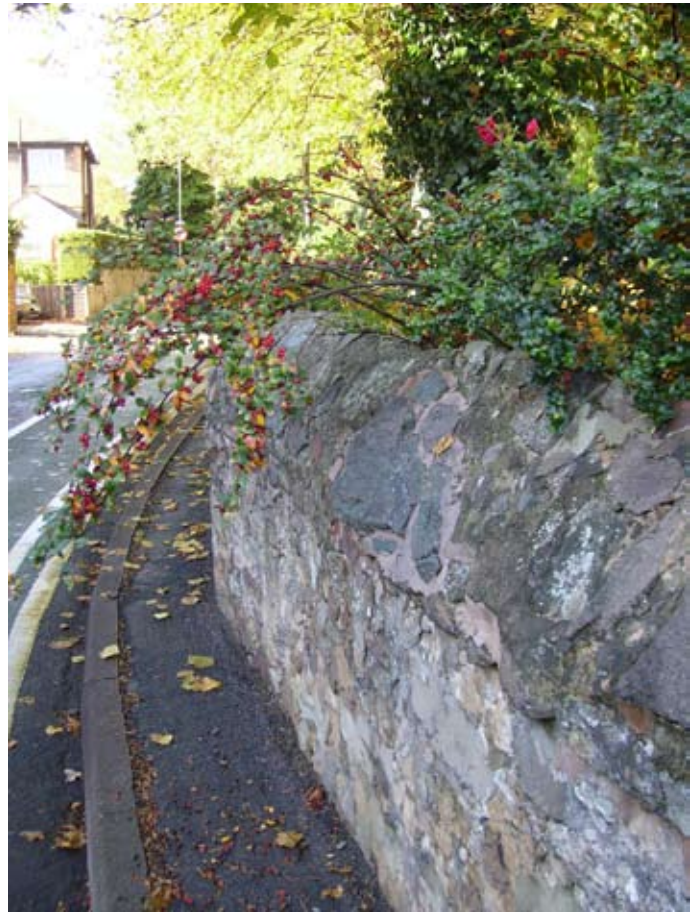
Granite boundary wall to St. Andrew's churchyard
