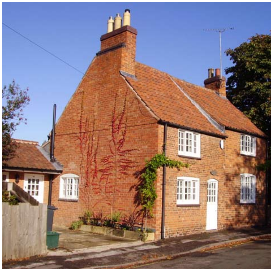
'Vine Cottage', 23 Old Church Street, is unique within the conservation area in having a red pantile roof.
