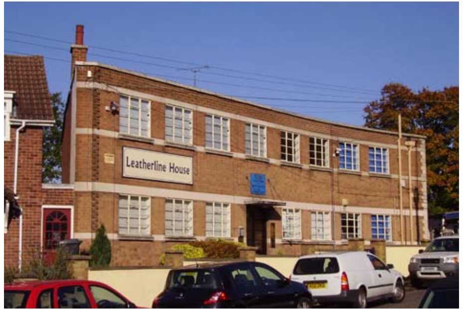
The former factory premises at 71 Narrow Lane has a curved façade; the original metal casement window frames still survive intact and are important architectural features to this pleasing building.
