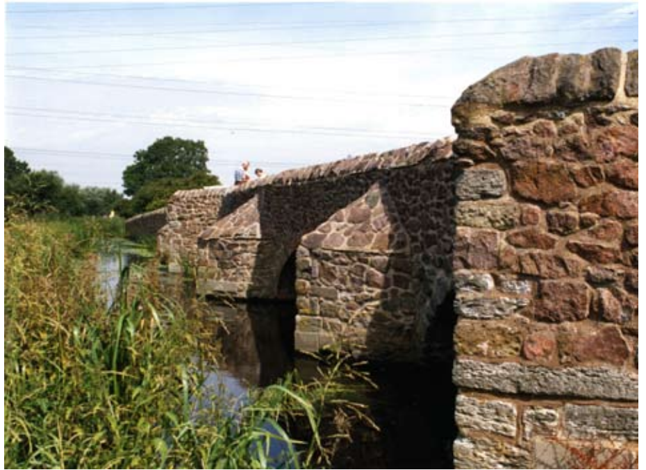
The Packhorse Bridge is a Scheduled Monument.
