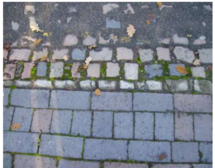
Old granite setts combined with original blue paviors provide texture and character to Old Church Street and other areas of the public realm within the conservation area.
