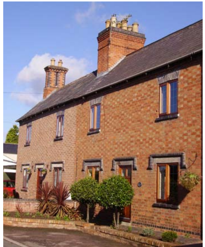
This pair of cottages at 27-29 Sanvey Lane incorporates some fine blue brick hood moulds above the window and the windows and sills.
