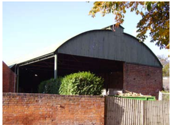
A detail of the old barn to Aylestone Farm, Sanvey Lane.
