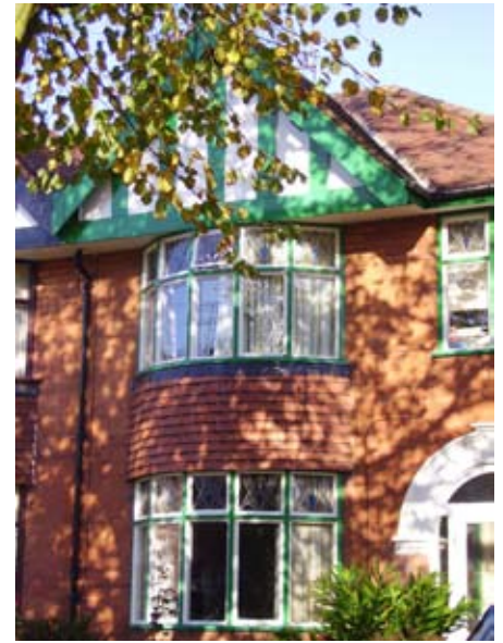
Above and left: Several of the properties in Croft Avenue retain their original attractive windows and doors and applied timber decoration to the gables.
