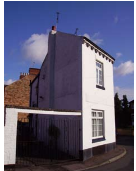
The corner property at 25 Sanvey Lane.
