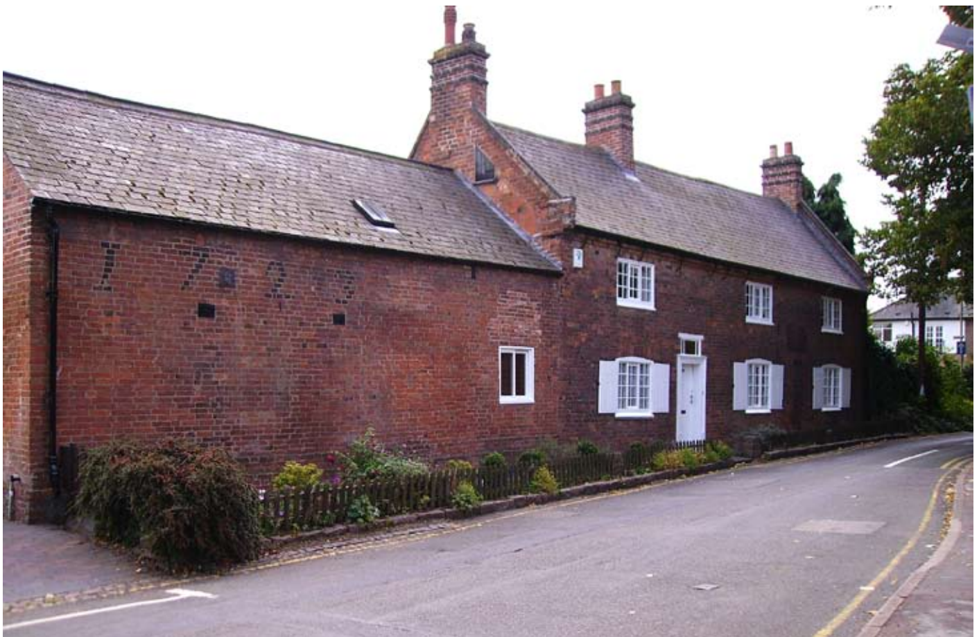
Number 90 Old Church Street is listed Grade II.
