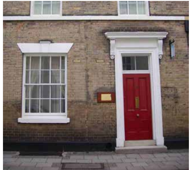
Pale bricks manufactured in Cambridgeshire were chosen for the small range of terraced houses at 18 to 28 Friar Lane.
