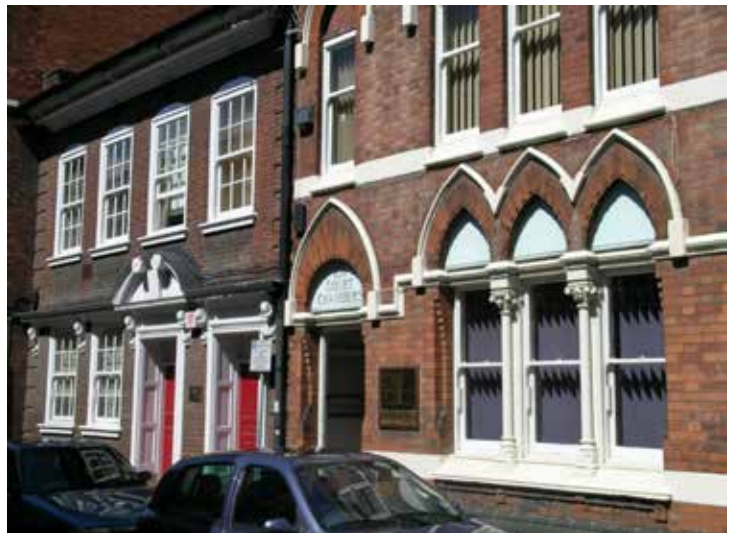
Court Chambers 27½ Friar Lane and adjacent at number 29, is a Queen Anne style brick building of 1904.
