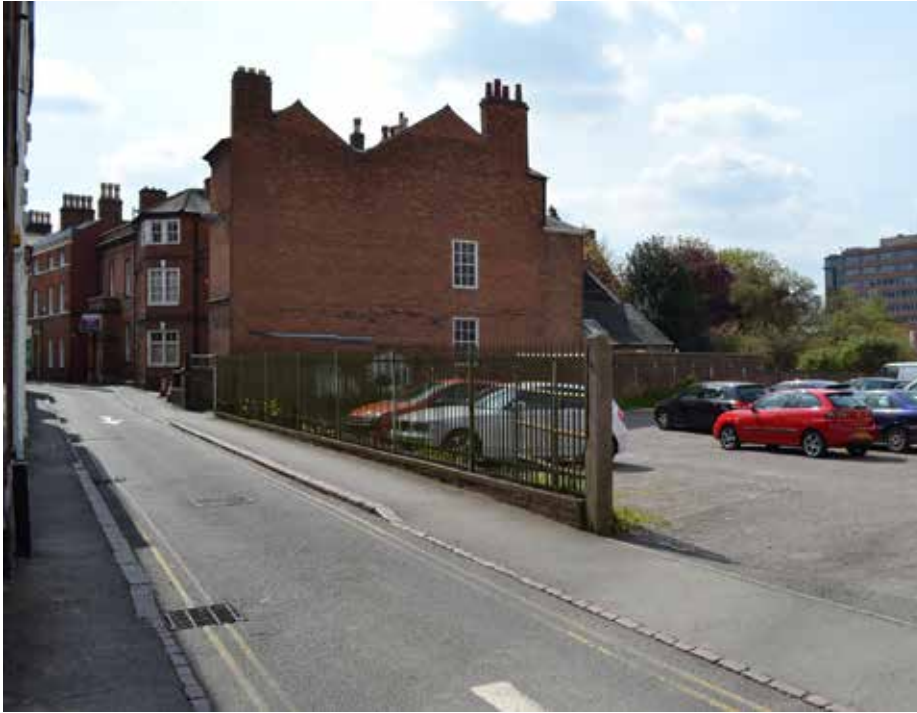
Poor boundary treatment of New Street Car Park
