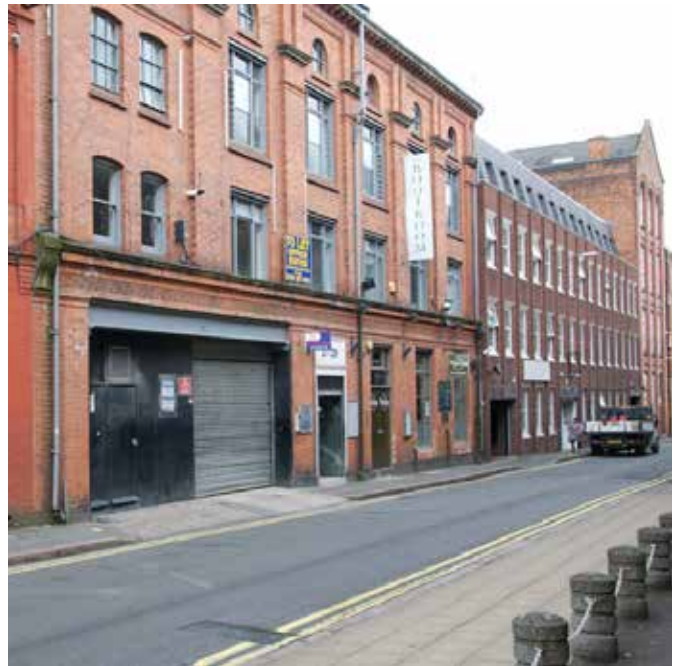
Modern offices sit alongside a converted Victorian factory on Millstone Lane.
