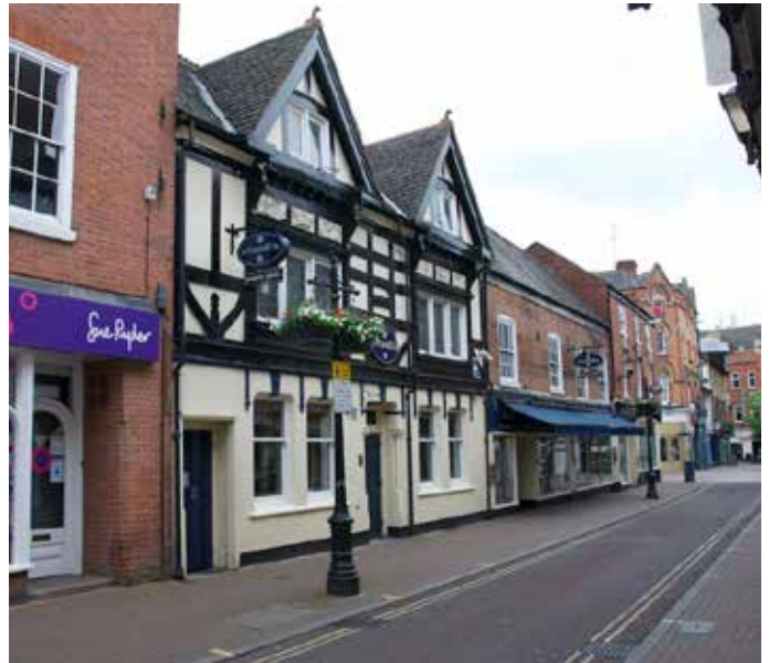
Loseby Lane: three storey brick 18th century former townhouses and adjoining the former Crown and Thistle public house of the 19th century with its heavy gables and mock timbering and plaster panels.
