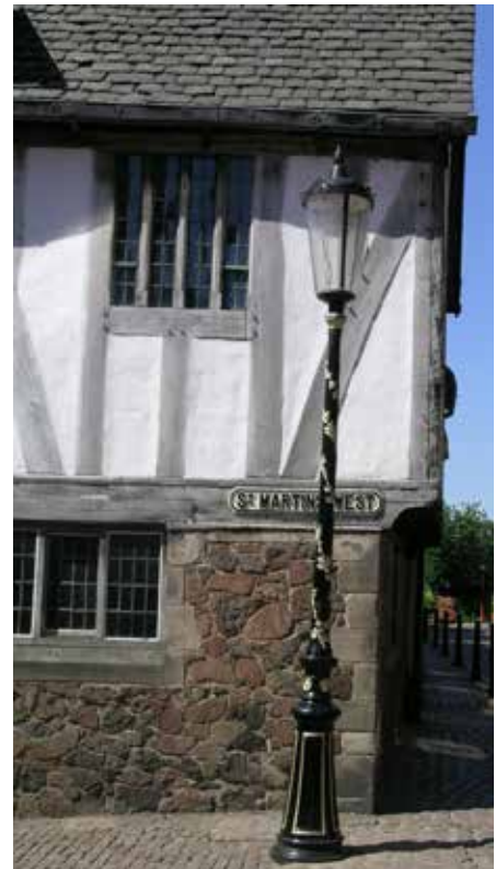
The Guildhall: the use of various building materials (timber, slate, stone, and cast metal etc) are important elements in giving character and texture to the conservation area.
