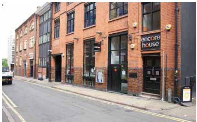
Victorian factories at 32 & 36 Millstone Lane.
