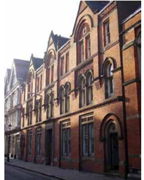
Conway Buildings, 7 Grey Friars, designed in the Gothic style by Stockdale Harrison.
