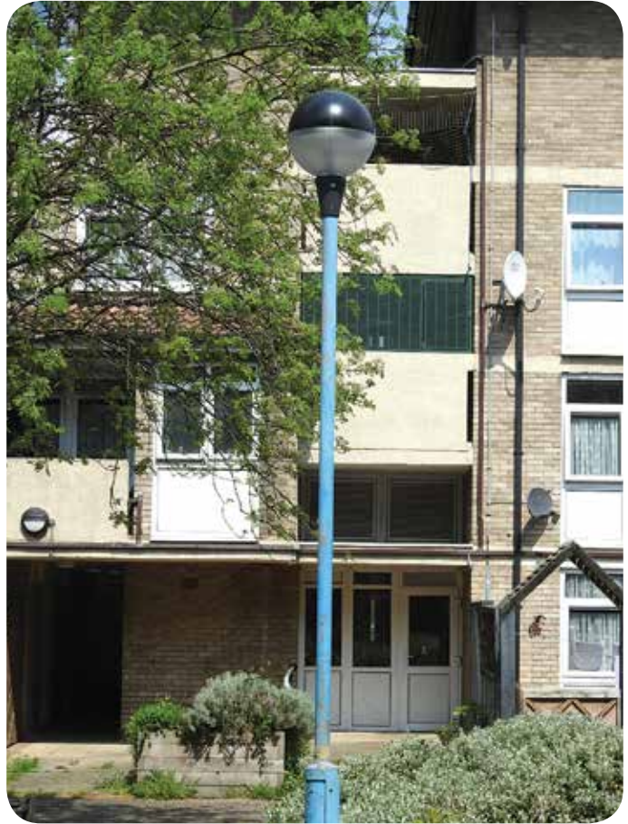
Communal area lighting at a council housing property
