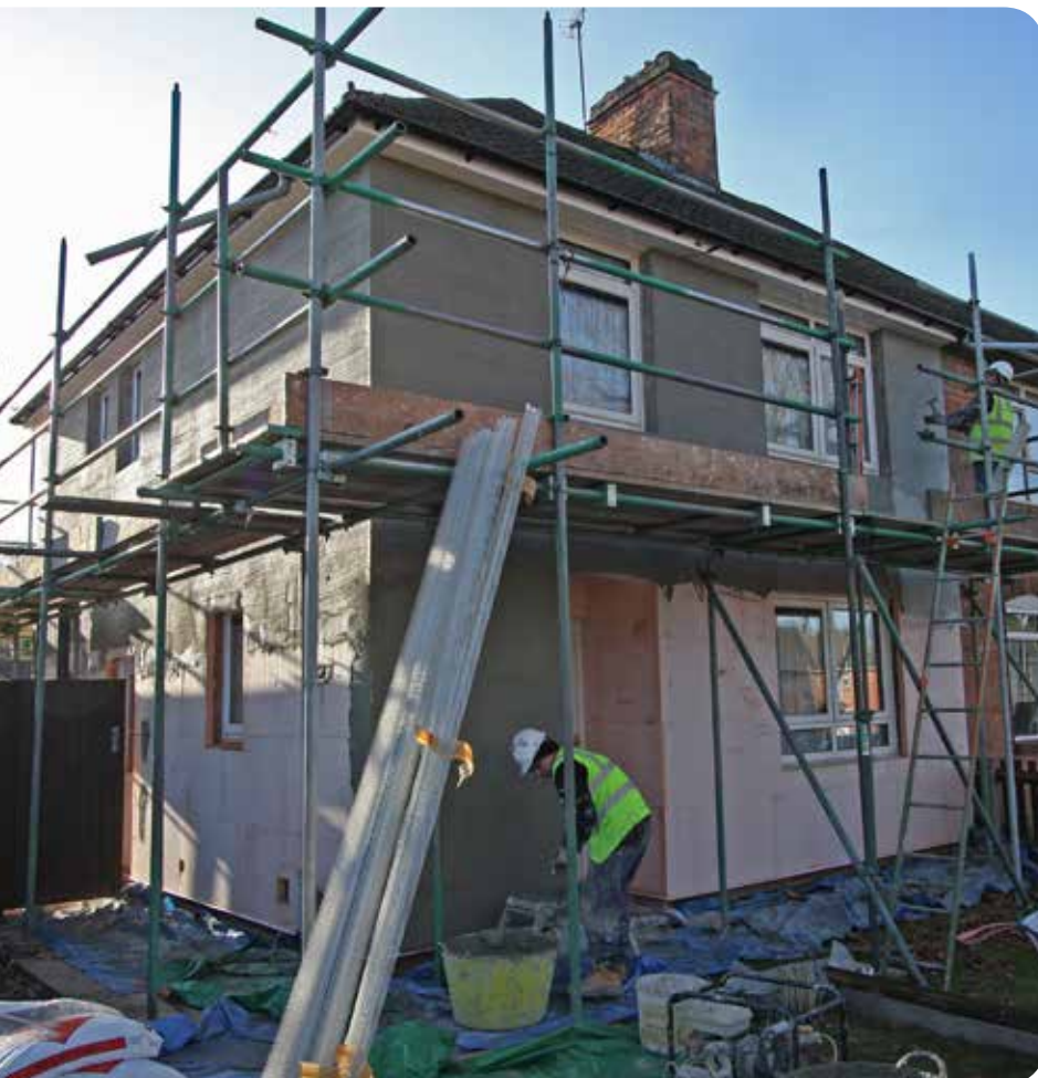
A house being fitted with external wall insulation
