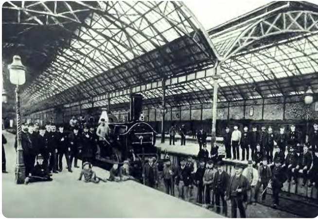
Figure 8: Belgrave Road Railway Station Opening 1882, Leicester County Council
