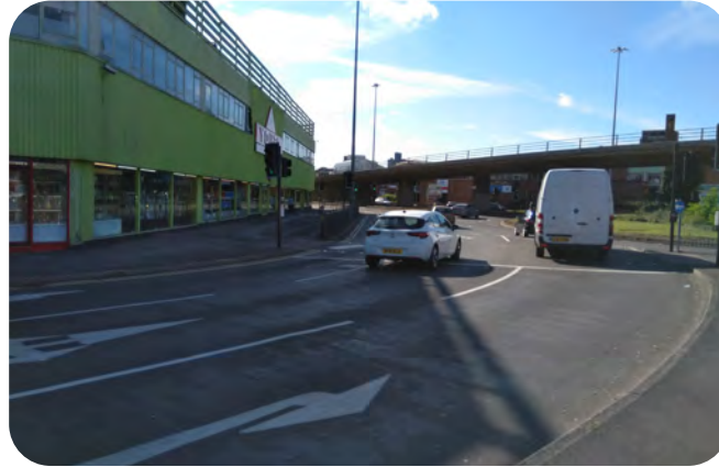
Figure 39: Ring Road, Burleys Way/ St Matthews Way
