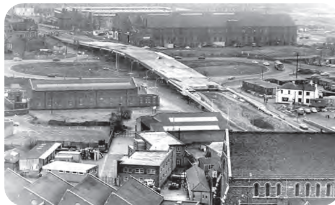
Figure 22: Construction of Belgrave Road Flyover 1973 (Leicester Mercury)
