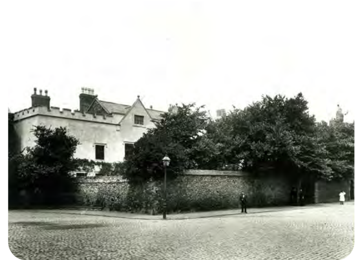
Figure 19: Chantry & Skeffington House with the Wall to the Newarke Still Standing. c1910 (Story of Leicester)
