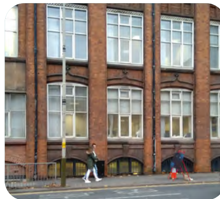
Windows and openings
