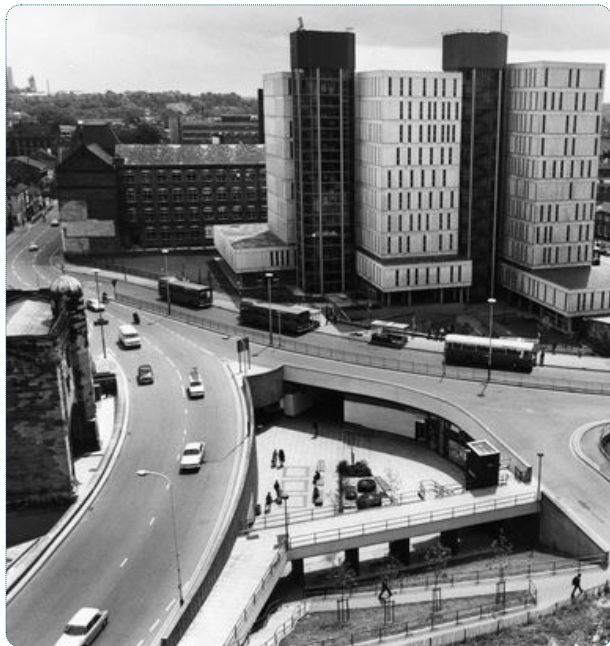
Figure 10: View South Showing The Newarke, Oxford Street, the James Went Building in 1974. (Leicester Mercury)
