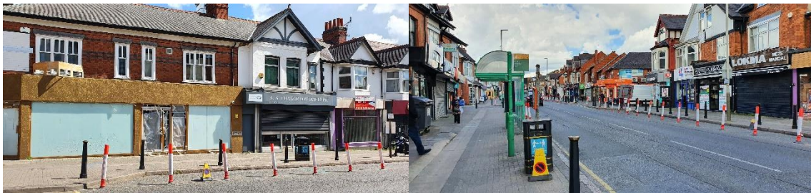
Figure 3: Refurbished unit, Evington Road
