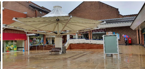
Figure 2: External Pedestrian Walkway
