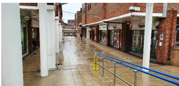
Figure 3: External Pedestrian Walkway
