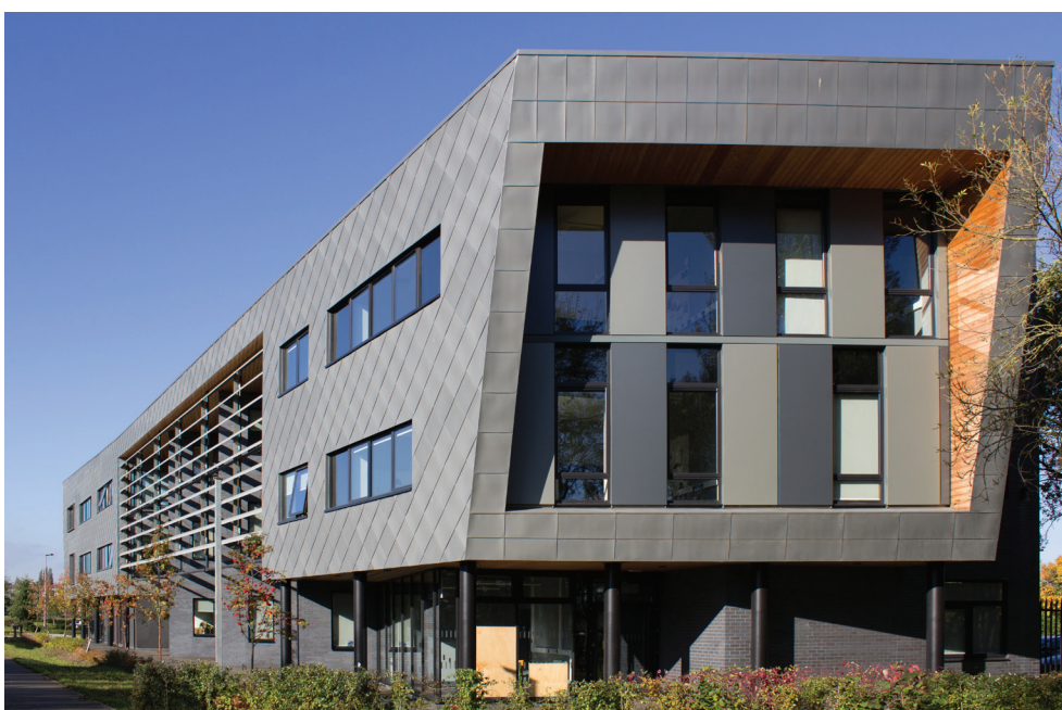
Dock Business Center
