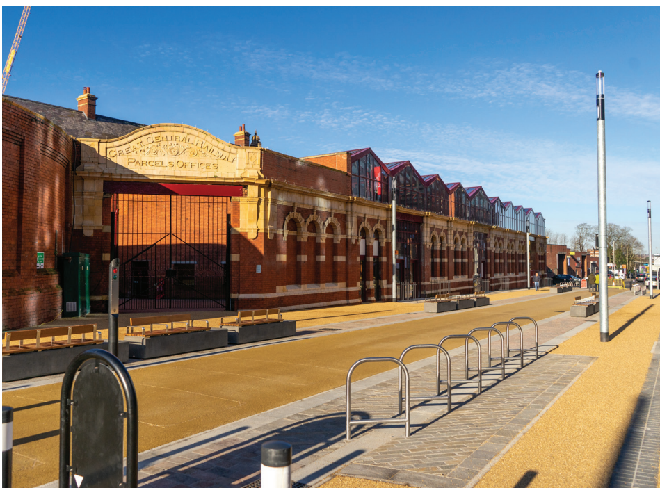
Former Great Central Station
