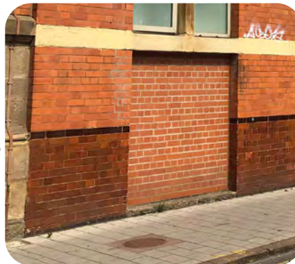
Glazed Brick Plinths
