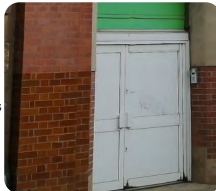
Glazed Brick Plinths
