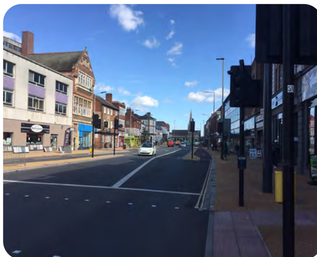
Figure 45: Improvements to Belgrave Gate
