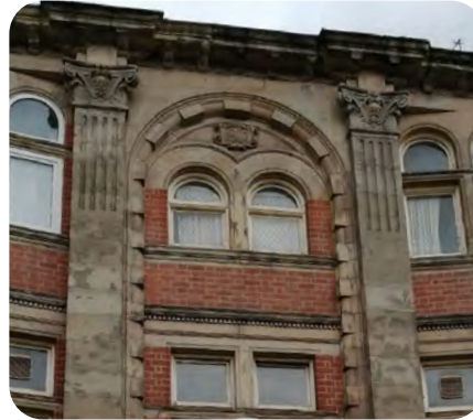
Arches - Doors & Windows
