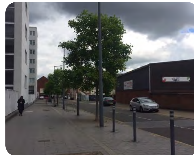
Figure 44: Wharf Street South Public Realm Improvements Secured with the Planning Permission for the Exchange Building
