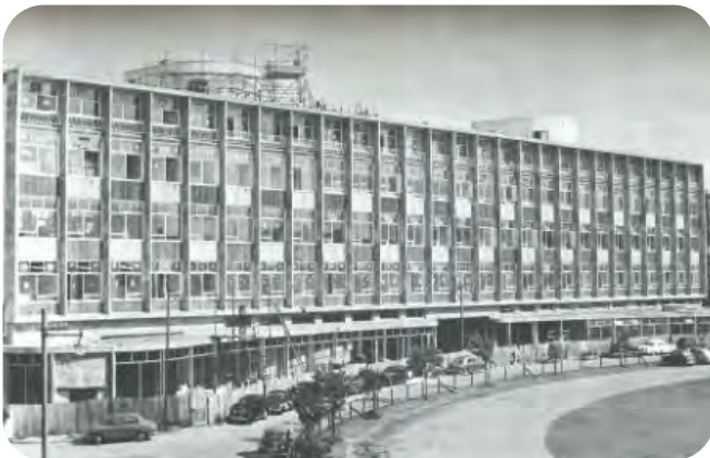
Figure 19: Leicester Telephone Exchange 1957 - Shops & Houses demolished to make way (© Leicester Mercury)
