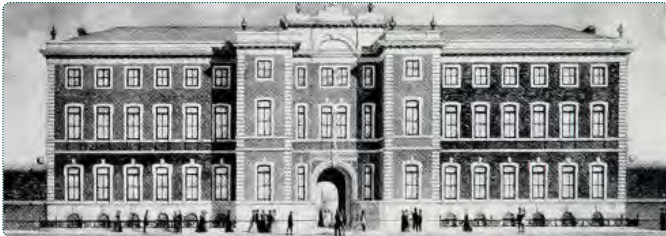
Figure 23: The 1865 Factory Building Designed by William Jackson
