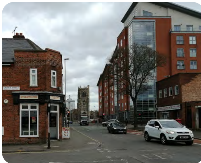
Figure 54: St. Margaret's Church from Sanvey Gate
