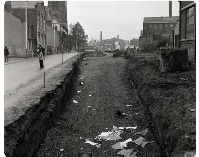
Figure 12: Construction of St. Margaret's Way, 1969
