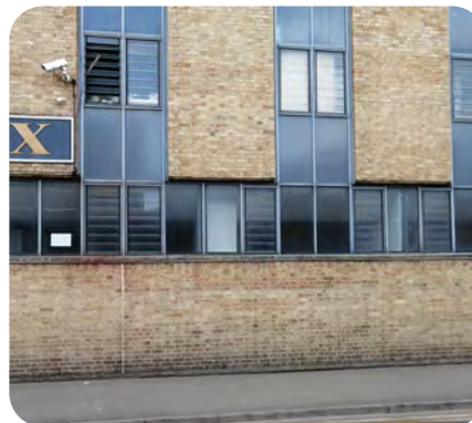
Framing of Windows
