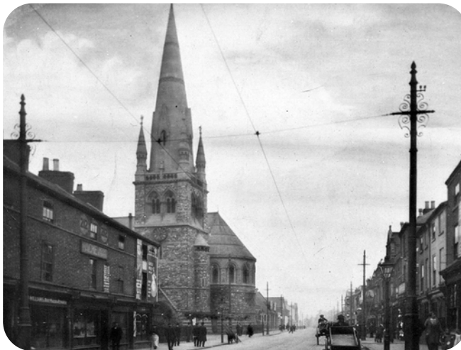
Figure 13: St. Marks Church, 1912 (De Montfort University)
