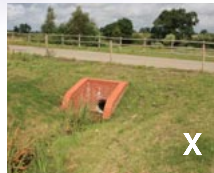
Picture of brick built headwall
