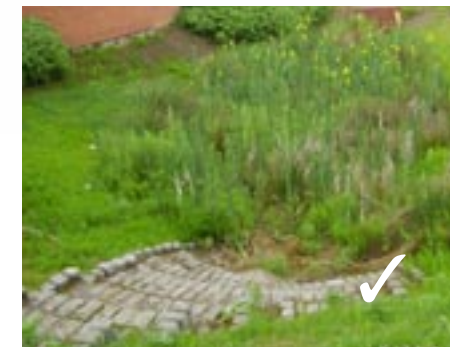
Picture of hard construction in line with the slope
