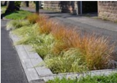
Retrofit highway rain garden on former verge
