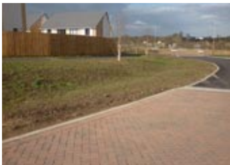
Adopted permeable block paving Damson Drive, Leicester
