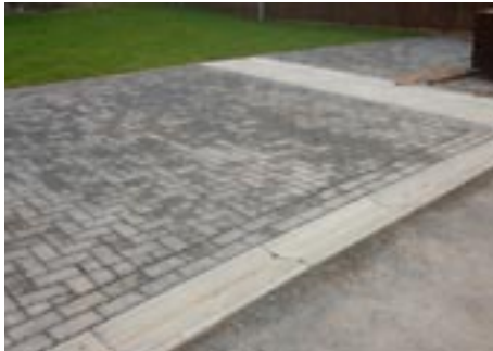
Parking area Dartmouth Gardens
