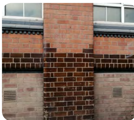
Glazed Brick Plinths
