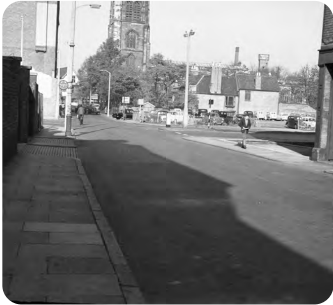
Figure 24: View Down Church Gate Towards St. Margaret's Church Prior to the Construction of Burley's Way (Leicester City Council)
