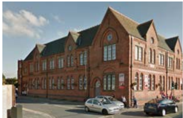
Slater Primary School - one of only two primary education institutions located within the CDA boundary, in the Waterside
