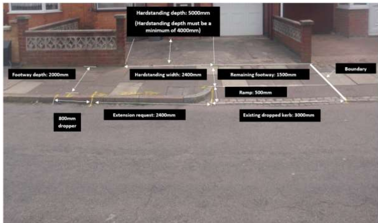
Photograph 2- Illustrating dropped kerb extension with dimensions
