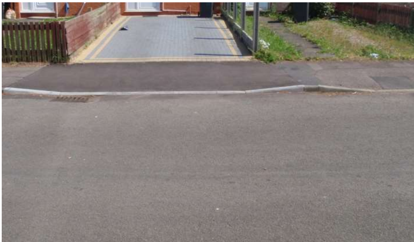
Example of a photo illustrating a completed hardstanding and dropped kerb
