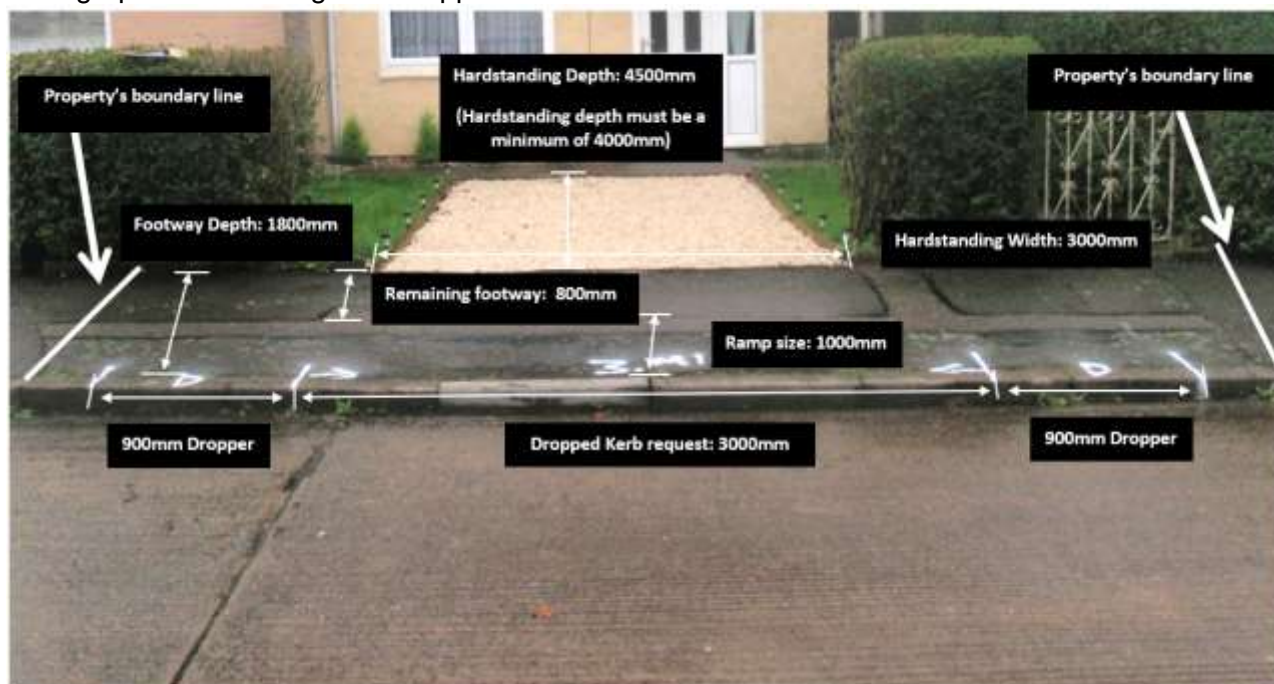
Photograph 1- Illustrating new dropped kerb with dimensions
