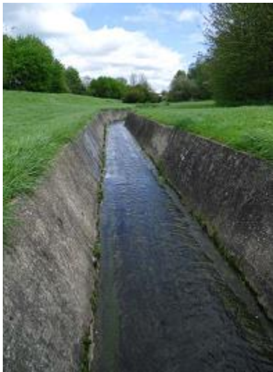
Figure 5.29: Channelled brook – Netherhall Open Space
