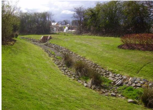
Figure 5.12: Swales Taking Water from Housing Areas to Main Water Courses
