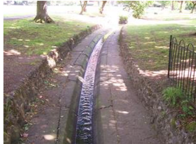
Figure 5.30: Channelled Section of Brook at Spinney Hill Park Pre-works
