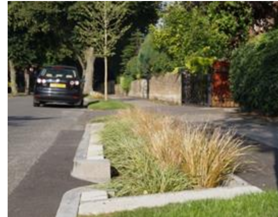
Figure 5.11: Road Verge Infiltration Trenches
