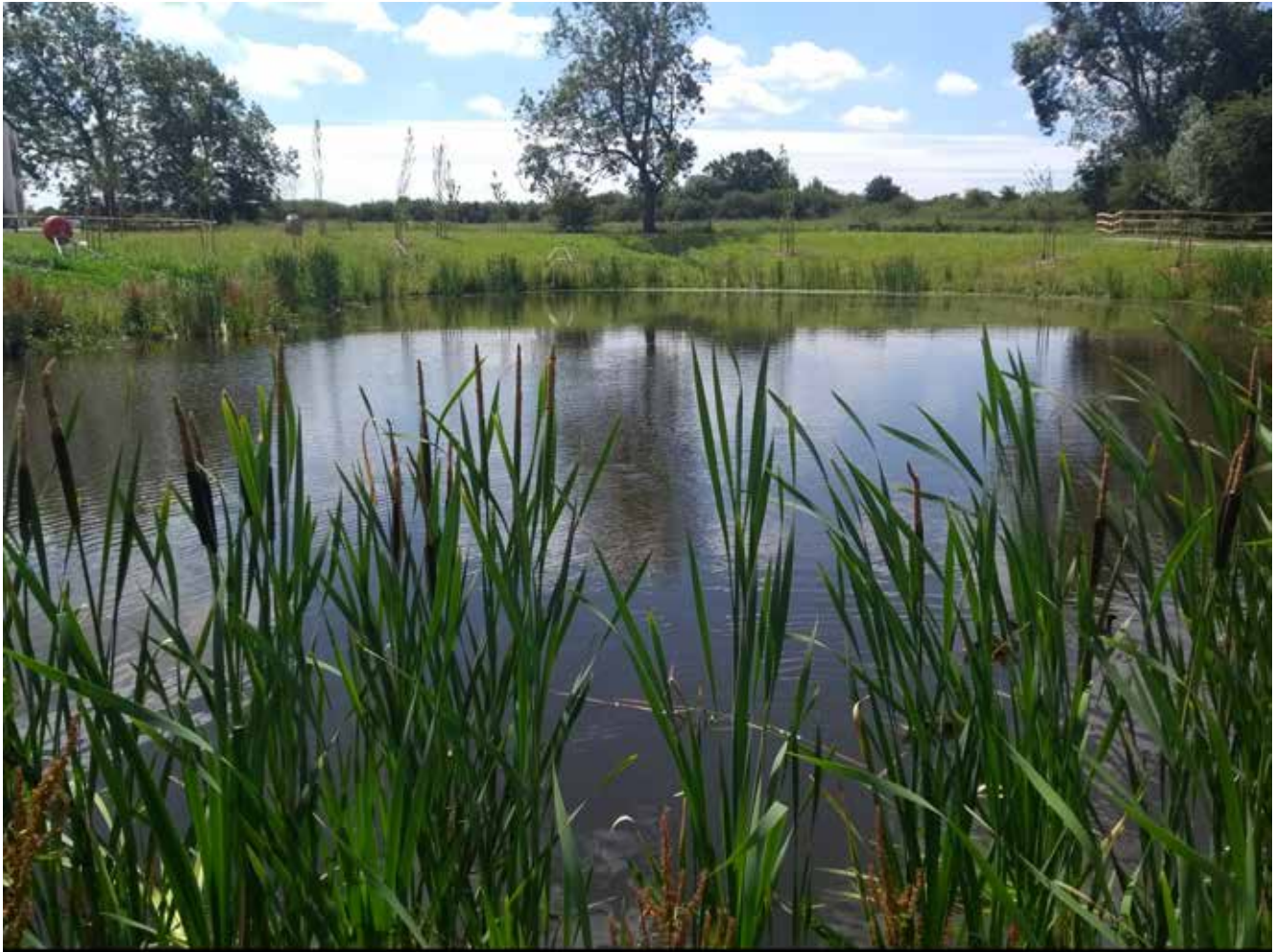
Sustainable urban drainage scheme at Ashton Green
