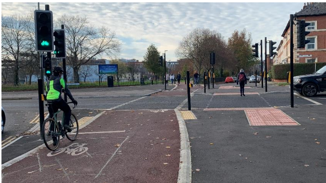
Tigers Way Crossing – with segregated pedestrians, cycles and vehicles
