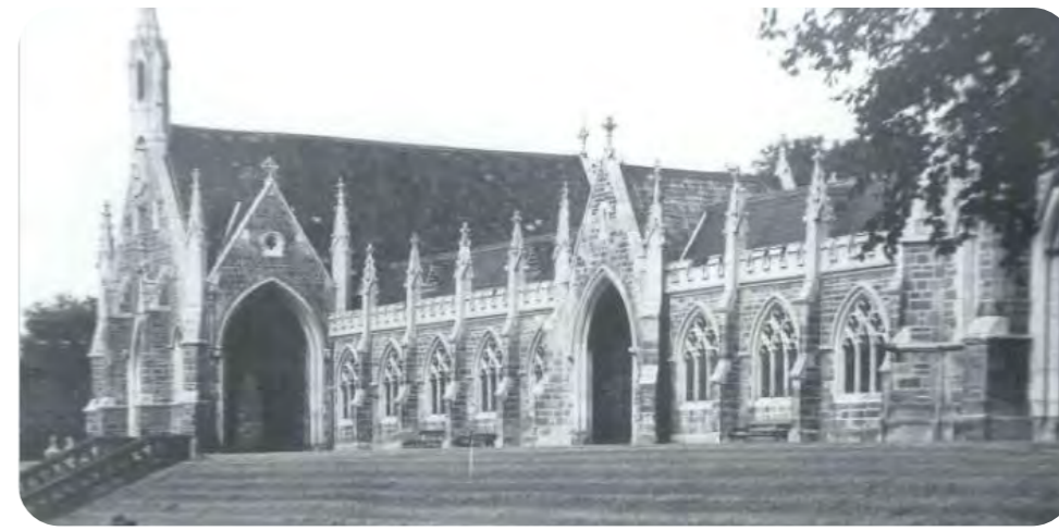
Figure 144. Welford Road Cemetery was opened in 1849. The chapel, placed on a elevated position was demolished in the 1960s (Malcolm Elliot: Leicester - A Pictorial History).
