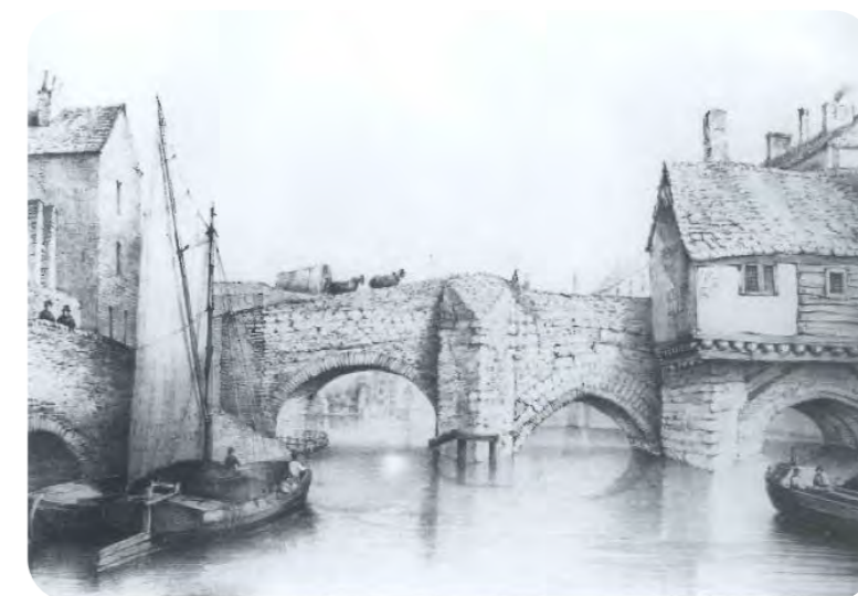
Figure 137. The old West Bridge from around 1841 (Malcolm Elliot: Leicester - A Pictorial History)
