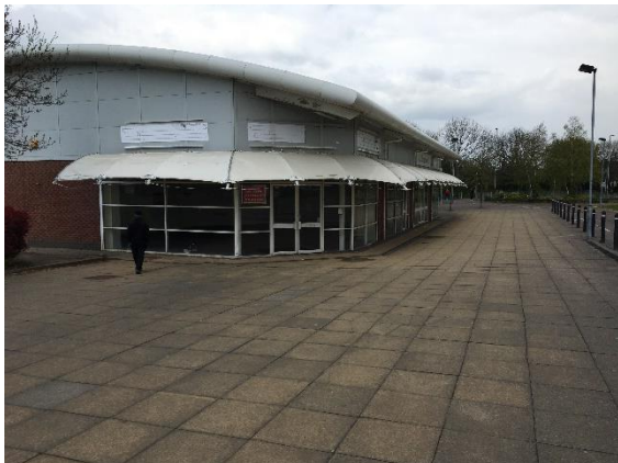
Figure 2: The eastern end of the local centre is focused on smaller retail units and community uses
