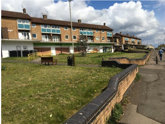
Figure 1: The retail parade is considerably set back from Thurncourt Road, and comprises ground floor retail with residential uses above
