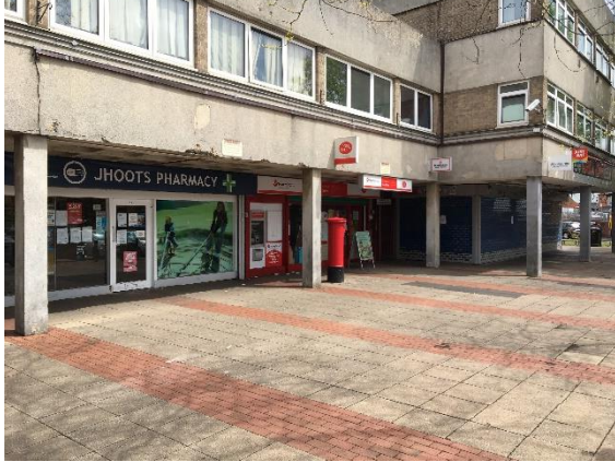
Figure 1: The retail parade of units adjacent to St Matthew's Centre
