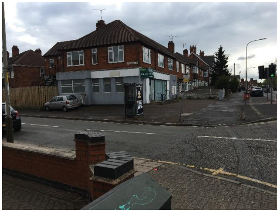
Figure 1: The vacant former TSB unit at the junction of Aylestone Road and Cavendish Road
