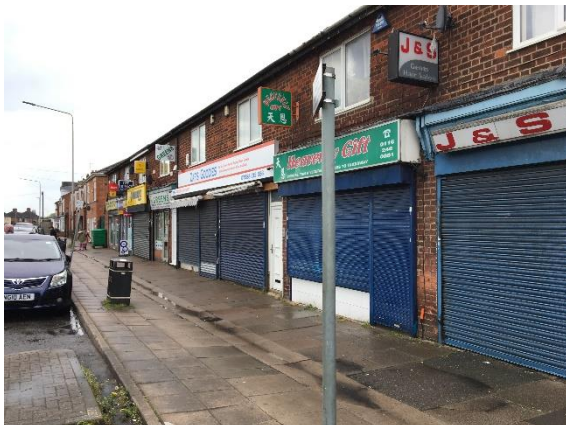
Figure 2: The retail units within the local centre are generally rather tired in appearance and could benefit from investment
