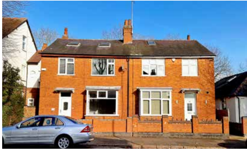
Pair of Edwardian Houses with no garages or off street parking
