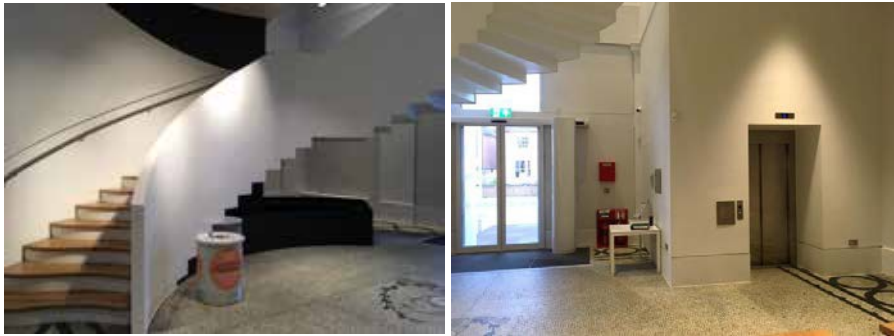
Foyer (Stairs & Lift)
